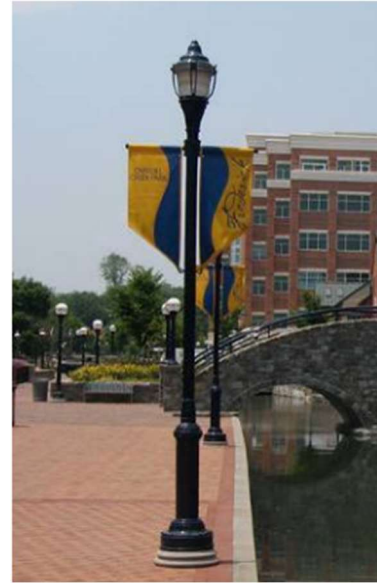
Streetlights should be designed to accommodate banners and associated wind loads on pole 4” minimum pole diameter.
