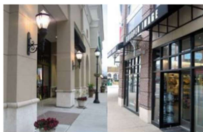
Traditional storefront entry design within modern day building techniques.
