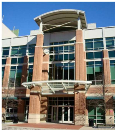
Canopy storefront with special structure treatment creates stronger focal point along the street front.
