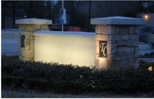
Well-hidden ground-mounted sign illumination.
