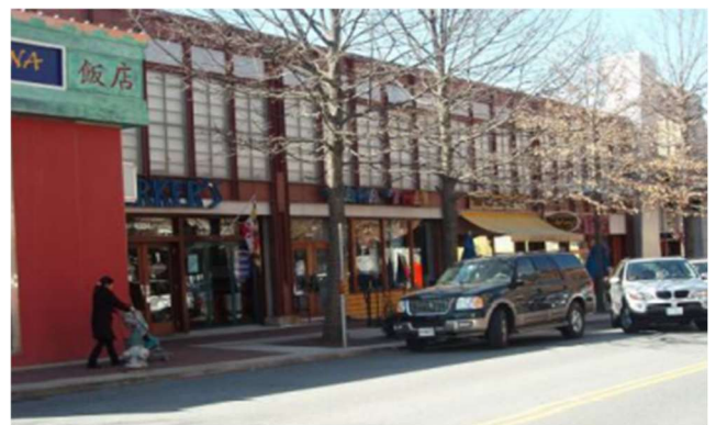
Exposed steel structure façades are not appropriate as a predominant building façade.
