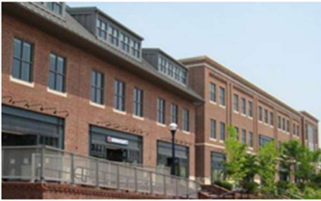
A pitch roof with dormer design proportioned to main structure of the
