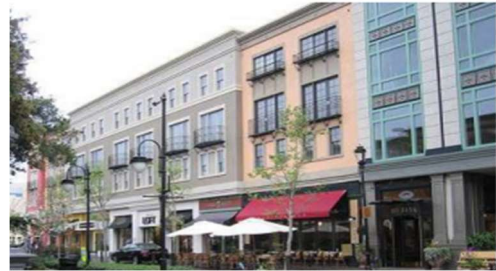
Consistency in window rhythm and scale can create visual harmony among individual structures.
