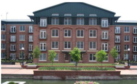
Proportionate symmetrical roof structure complements the overall symmetrical building form.
