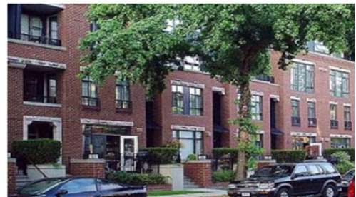
Change of window type and size can be designed to help break the building mass and animate street life.
