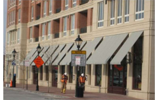
Awnings extended to cover sidewalks provide shading.
