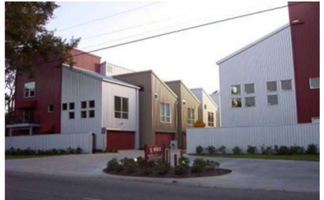
Corrugated Metal siding is not appropriate as a predominant building façade.
