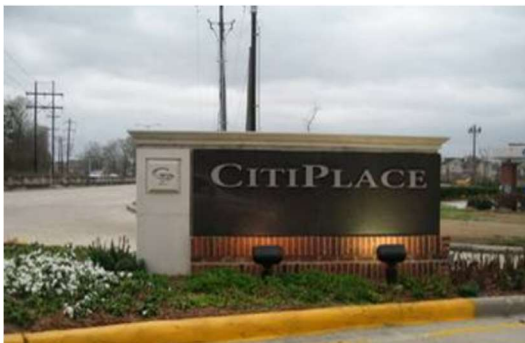
Poorly hidden ground-mounted sign illumination
