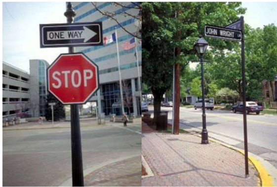
Grouping of standard regulatory signs adapted to allow use of ornamental fluted poles, frames, and post cap.
