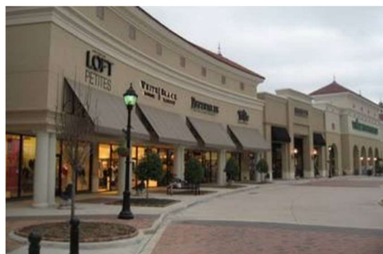
Complementary facade signs installed within the commercial tablatore.
