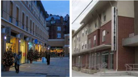
Traditional & contemporary mixed-use building with large storefront and smaller residential windows.
