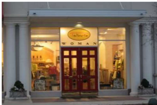
Good example of window transom signage.
