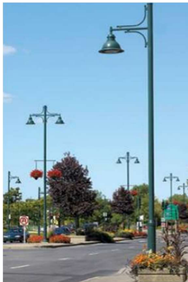
Traditional Style streetlight fixtures designed with accessory arms to accommodate hanging planters- 20’ height with full cutoff.
