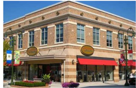
Flat roof and parapet treatments with cornices and trims are appropriate for
