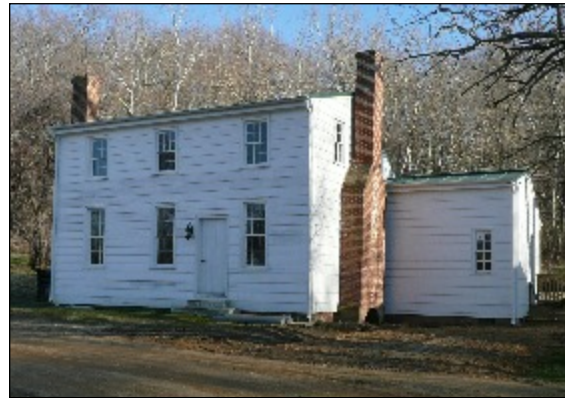
Figure 9: Recently restored Burch House (Catslide)
