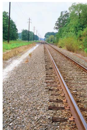
The Conrail line near White Oak Road, looking south
