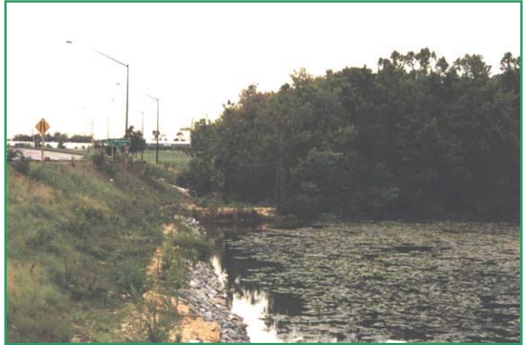
Storm water management pond serving the US 301 MD 5 intersection at the northern edge of the Sub-Area.
