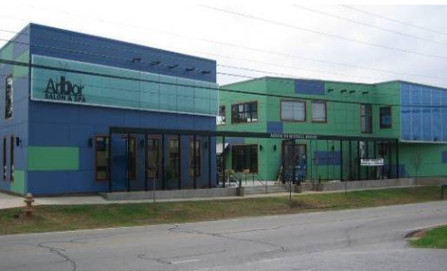
Sheet Aluminum or metal cladding façades are not appropriate as predominant building façade
