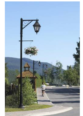
Traditional style streetlight fixtures designed with accessory arms to accommodate hanging planters – 20’ height with full cutoff
