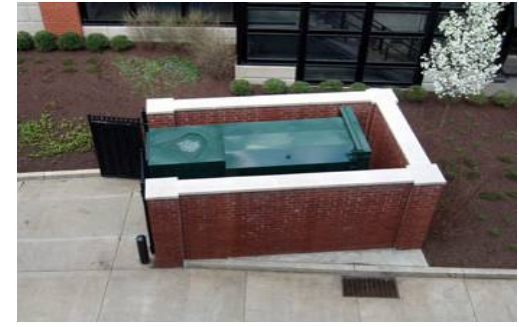
Example of recycled materials compactor screened by masonry enclosure
