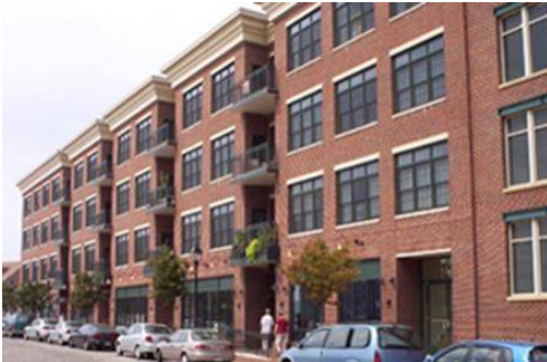
Example of change of building material and window types as a transition
