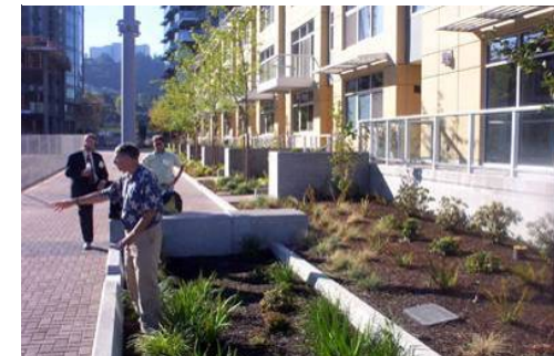
Green street techniques to filter stormwater before entering storm sewer system
