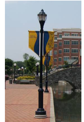
Streetlights should be designed to accommodate banners & associated wind loads on pole 4” Minimum pole diameter
