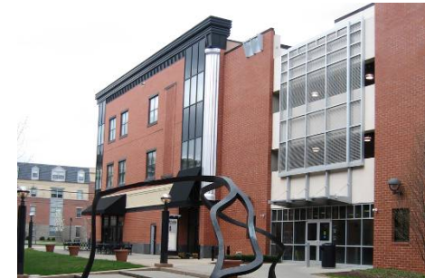
Integrated parking structure façade designed to be compatible with the main structure design and material
