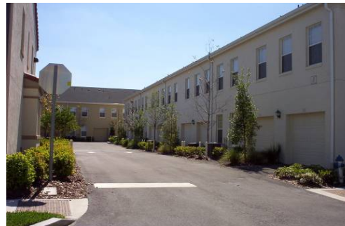
Example of inadequate residential rear façade treatment along an alleyway
