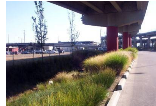
Bio-swale use in parking lots to filter pollutants from stormwater prior to entering storm sewer system
