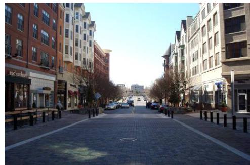
Urban Major Collector streetscape with special pavement at major crosswalks
