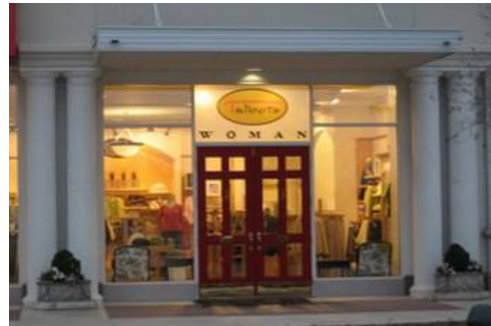
Good example of window transom signage
