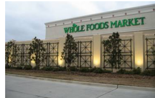
Common service area screened from view with fenestrated wall, plant materials and accent lighting
