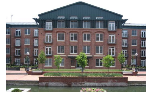
Proportionate symmetrical roof structure complements the overall symmetrical building form
