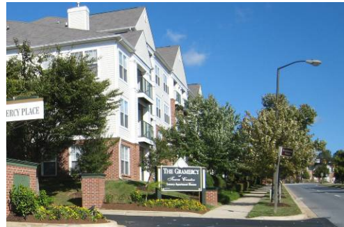
Urban Local Road treatment with patterned / scored concrete walkways and continuous lawn panels
