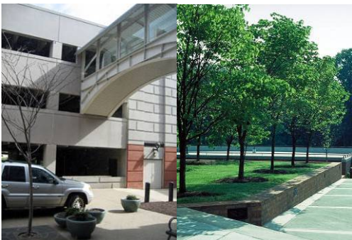
Example of pedestrian bridge and roof top garden on integrated structured parking
