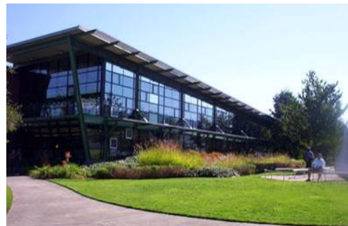
Perimeter rain gardens capture building stormwater run-off and re-use for natural irrigation
