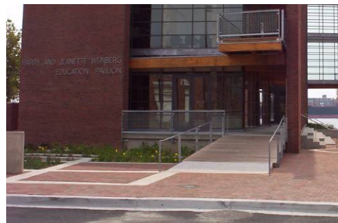
Good example of building accessible ramp compliant with ADA standard
