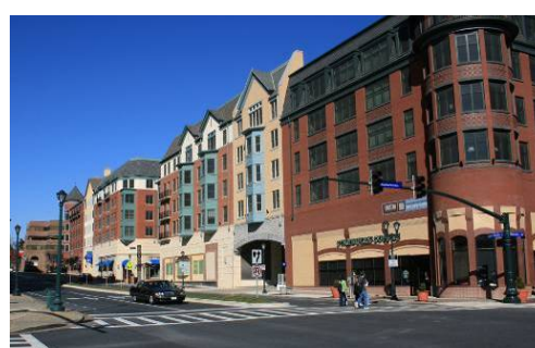
Variety in roof treatment provides visual interest to the skylines & fenestrates the monotonous facade
