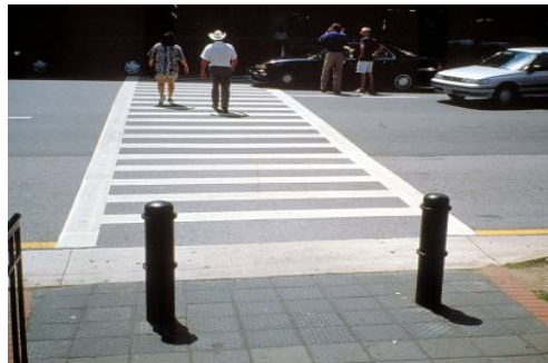
A crosswalk striped with paint or thermoplastic vinyl tape
