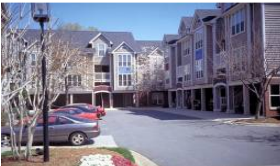
Example of integrated garage on the first floor of the building accessing from the rear and/or side
