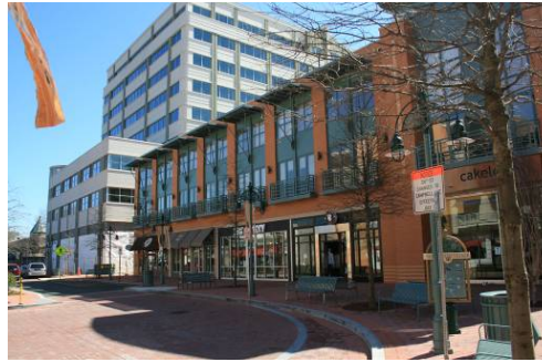
Example of façade articulation
