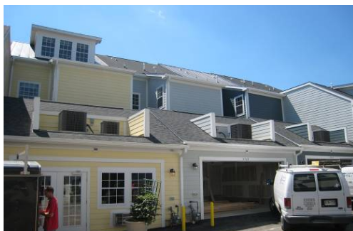
Exposed air conditioning unit in residential building can simply be treated with additional railing/screen
