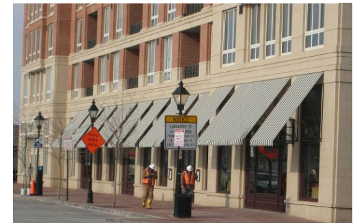
Awnings extended to cover sidewalks provide shading
