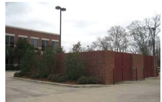
Good example of service area enclosure
