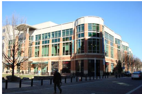
Example of façade articulation
