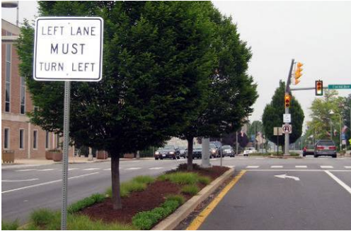
Urban Major Collector streetscape with well-sized median at intersection; would be appropriate for Acton Lane and Leonardtown Road intersections
