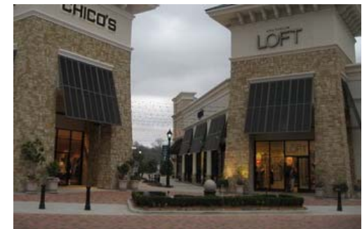
Shutter-like awning designs add variety to building textures & create sophisticated building character
