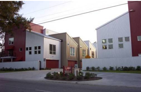
Corrugated Metal siding is not appropriate as a predominant building façade
