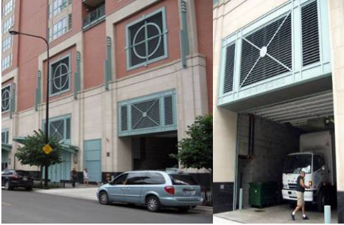
Sample service dock area built within larger scale structure
