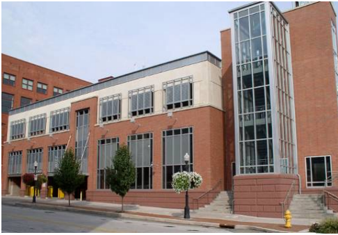
Good example of façade treatment where parking structure fronts the street
