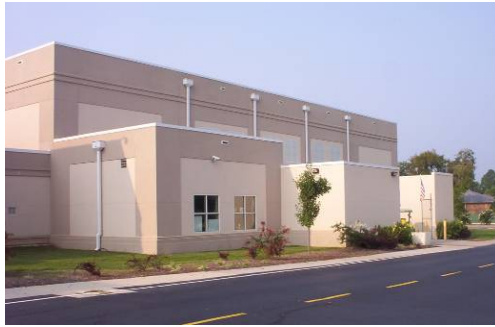
Exterior venting shafts and fume hoods should be screened from public view
