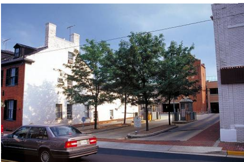
Shade trees screen the setback entry of an interior block parking structure
