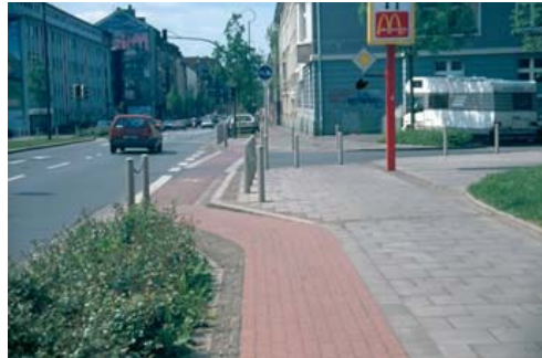
Bike lanes designated by special material such as color pavers are encouraged
