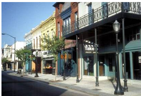
Decorative metal arcades and balconies
