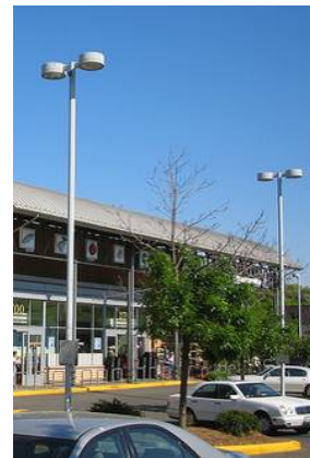
Traditional "shoebox" sharp cut-off parking lot lighting – 20' Maximum Height
