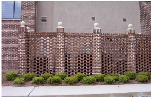
Vented brick wall screens a service area from the pedestrian walkway
