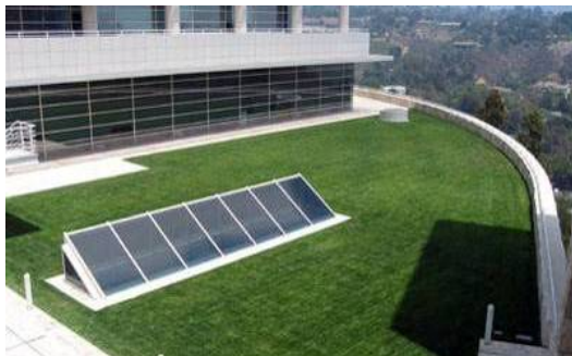
Turf-based green roof design with skylights to allow natural light to lower levels
