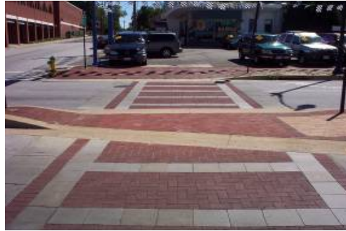
High-quality, pedestrian gateway crosswalk installation near the Naval Academy Campus - Annapolis, MD
