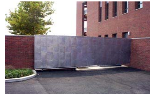
Sample contemporary style service enclosure using brick and galvanized metal slide gate panel
