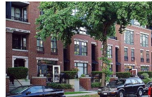
Change of window type and size can be designed to help break the building mass and animate street life
