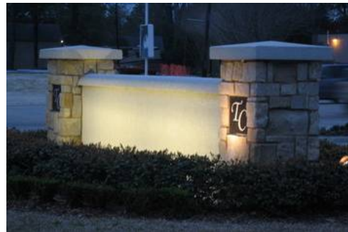
Well hidden ground-mounted sign illumination
