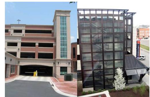
Elevator/stair towers and pedestrian entryways should be emphasized in the architecture to provide façade articulation in the parking structure
