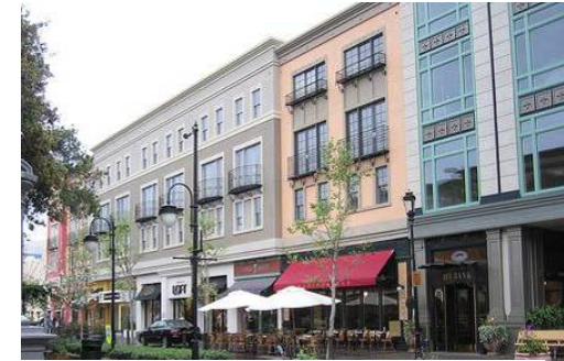
Consistency in window rhythm and scale can create visual harmony among individual structures
