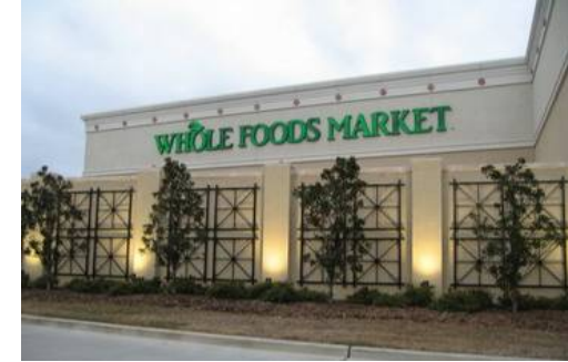
Good example of direct burial up-light illumination
