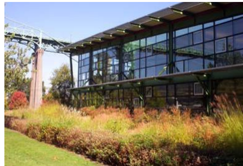
Cantilevered sun shades on windows to take advantage of natural lighting while regulating passive solar heating
