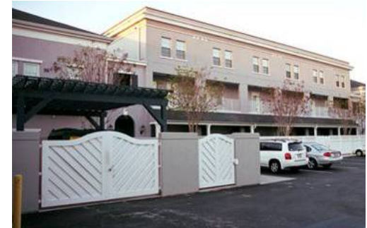
Example of stucco trash enclosure with ornamental doors and trellis to screen facility from resident views
