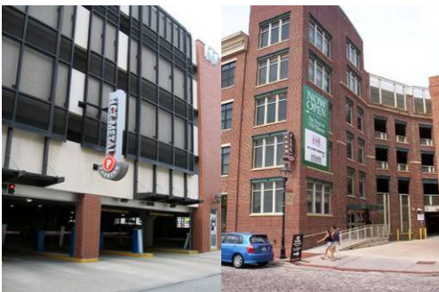
Parking garage entrances should have adequate way-finding signage
