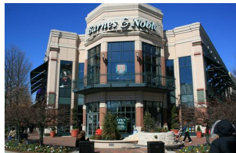
Recessed store front entry addresses the corner of public streets and creates public space use
