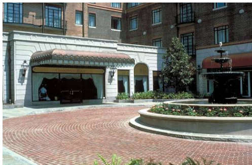
Arrival courtyard designed with special paving and water feature creates an urban plaza character
