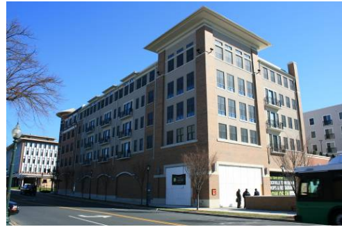
Example of inadequate rear façade treatment along a main road
