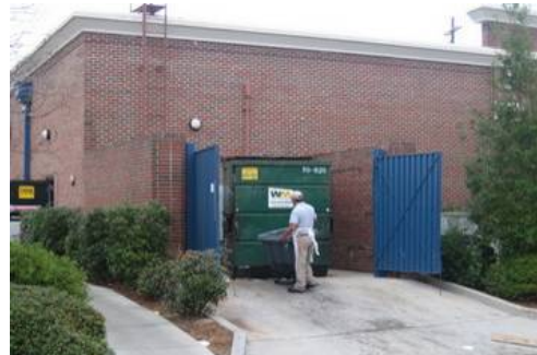
Example of trash enclosure with masonry wall & steel swing gates compatible with primary building facade
