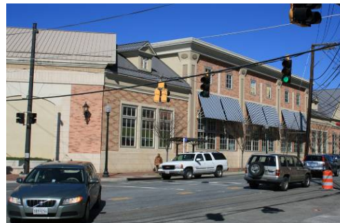
Appropriate use of different roof treatments helps break the building mass in specialty store use
