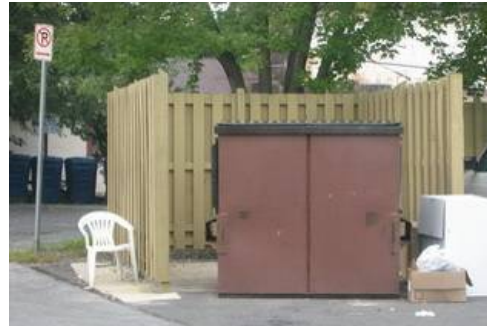
Trash containers must be visually screened on all sides from pedestrian and main vehicular paths
