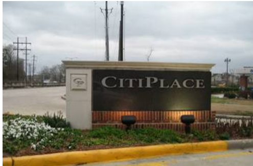
Poorly hidden ground-mounted sign illumination
