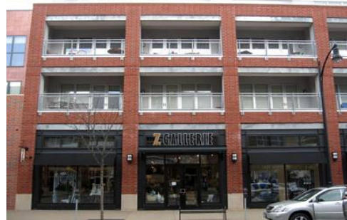
A hierarchy of windows and doors at both the lower & upper level creates symmetry
