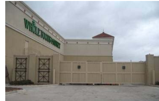
Good examples of common service area screened from view with fenestrated wall and gates
