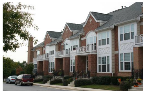
Balconies for residential building should be adequately sized for use, but not be used for outdoor storage
