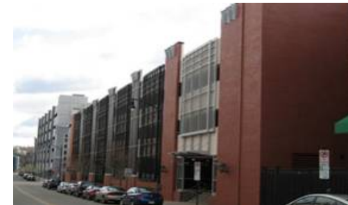
Façade screening panel designs serve as screening devices and add visual interest
