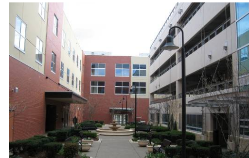
Example of good rear façade facing parking structure articulated with building color, canopy & landscaping
