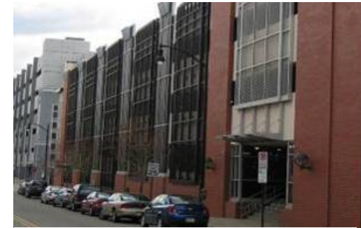
Example of façade articulation
