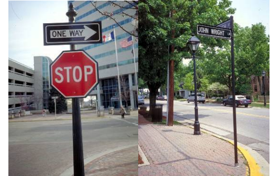
Grouping of standard regulatory signs adapted to allow use of ornamental fluted poles, frames and post cap
