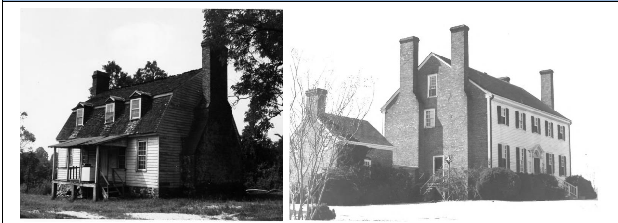
Figure 4.3.3-1: Images of Maxwell Hall (Left) and Rose Hill (Right) (NPS, 1974; NPS 1973)
