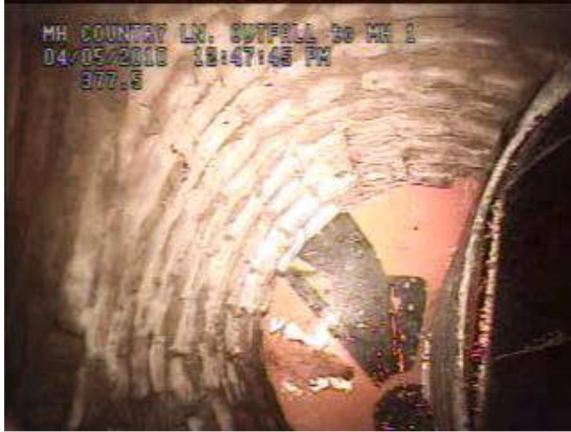
Photo 1 – 48” CMP – Buried Manhole
