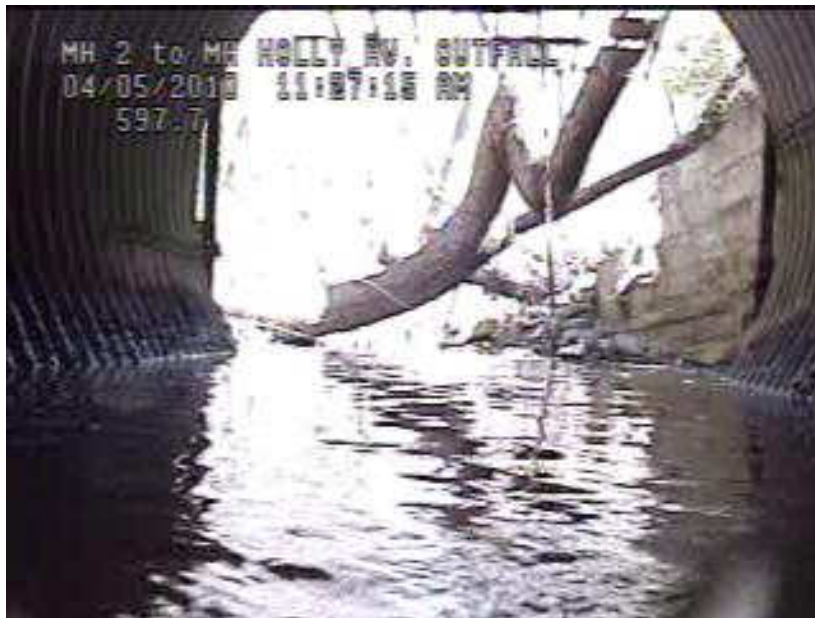
Photo 6 – 72” CMP – Pipe Outfall
