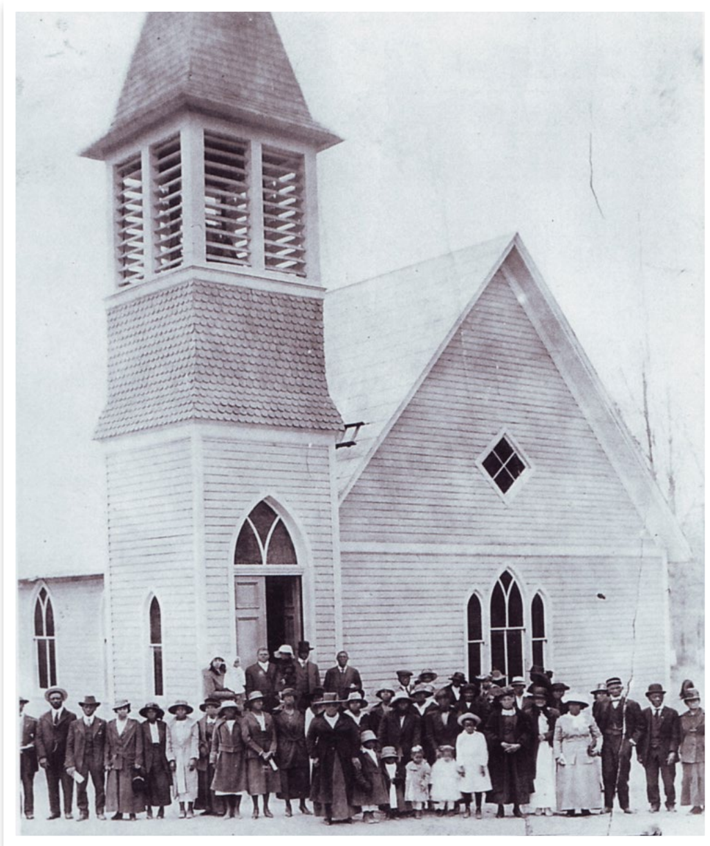
Built in 1910, the former United Methodist Episcopal Church was an important landmark in the village.
