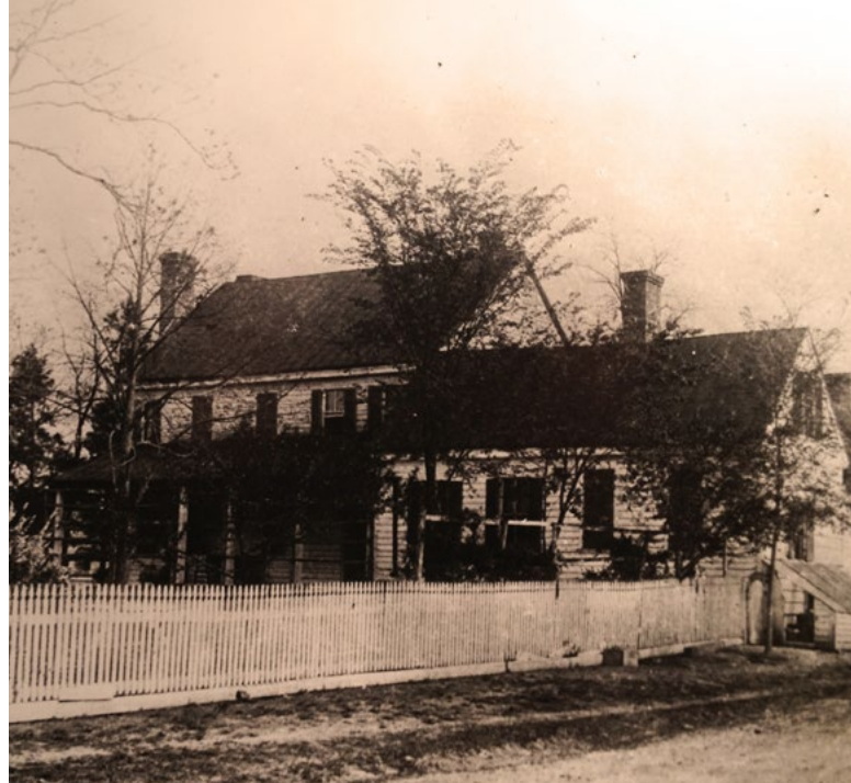
1901 photograph of Rich Hill that shows the existing row of outbuildings which have since been demolished. Photo by Osbourn Oldroyd.
