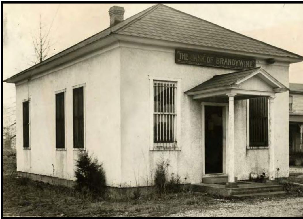
The Southern Maryland German American Bank was built in 1912 and later renamed the Bank of Brandywine (14110 Brandywine Road). The bank facilitated purchasing and reselling land to German immigrants through southern Prince Georges and northern Charles County. Photograph courtesy of Franklin A. Robinson, Jr.
