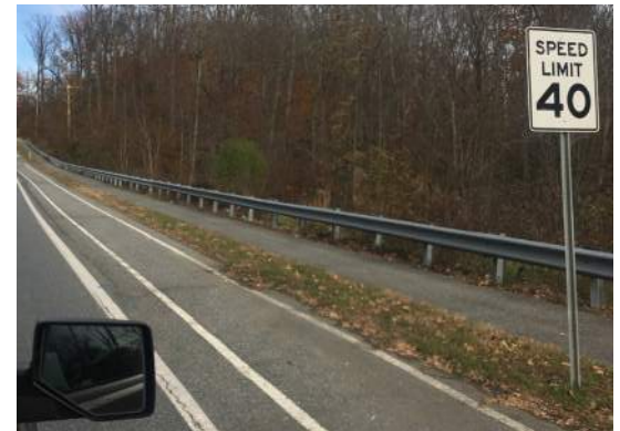
Even if facilities exist, few people will choose to bicycle if they are required to do so adjacent to high-speed traffic.
