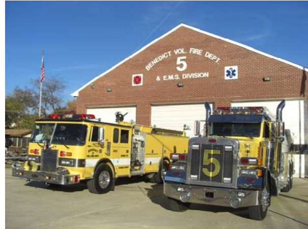
Fig. 2-14 – The existing firehouse
