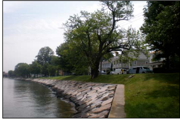
Fig. 2-27 – Example of structural erosion control on a shoreline
