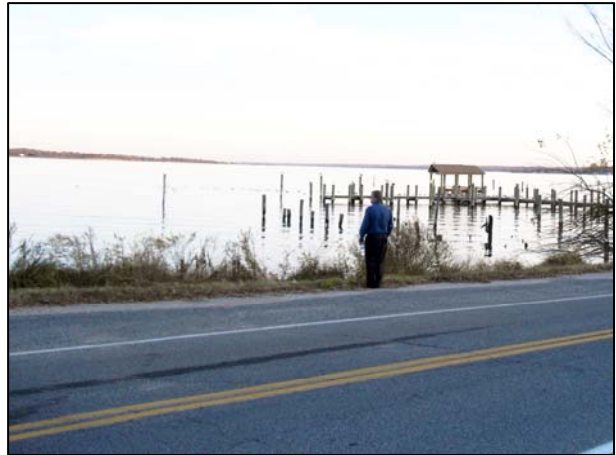
Fig. 2-18 – Along the waterfront, pedestrians walk on the asphalt shoulder of Benedict Avenue.
