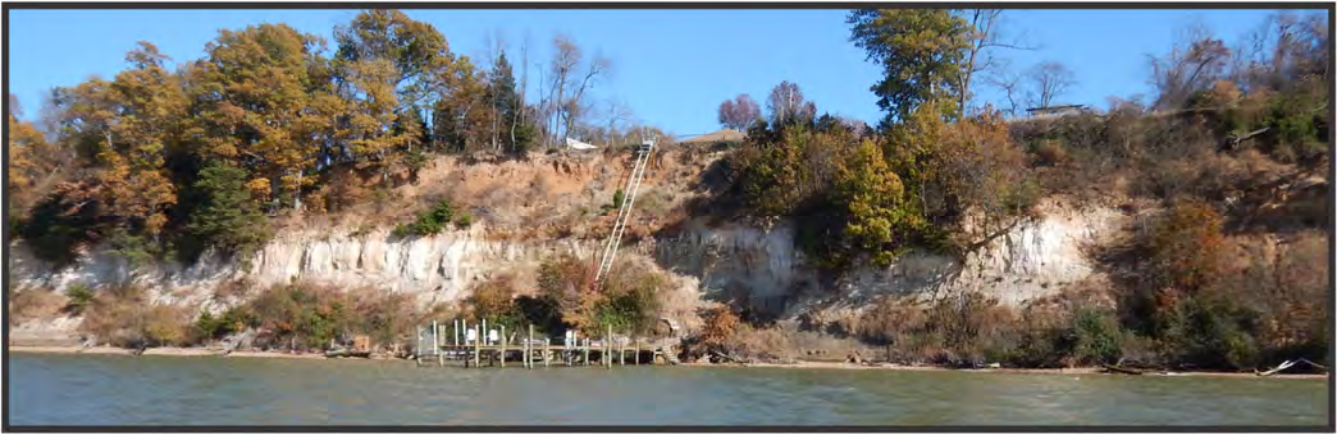
Figure 7-2. High eroding upland bluffs along Clifton, Site 66, recommend Type 5 sill.
