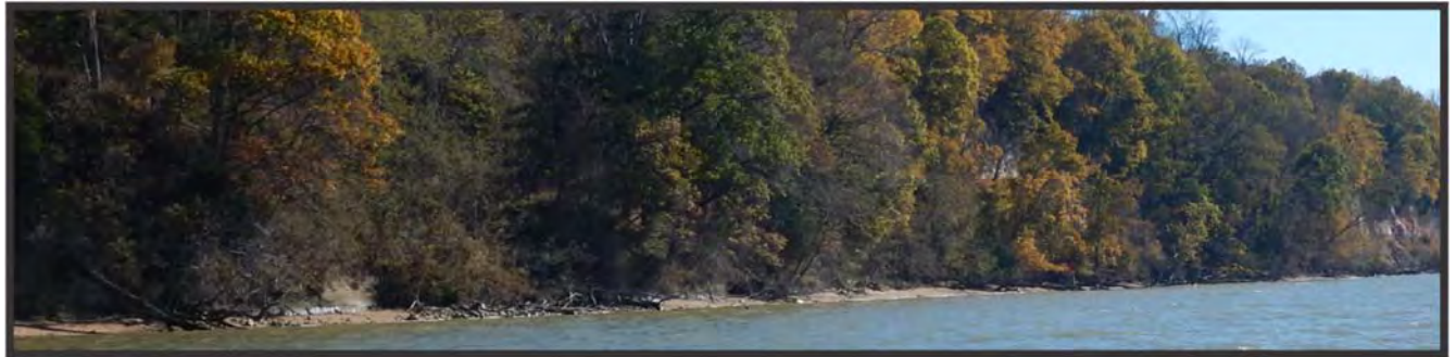
Figure 7-4. Eroding high upland bluffs with intermittent slumps. Site 73, recommend a Type 4 sill.
