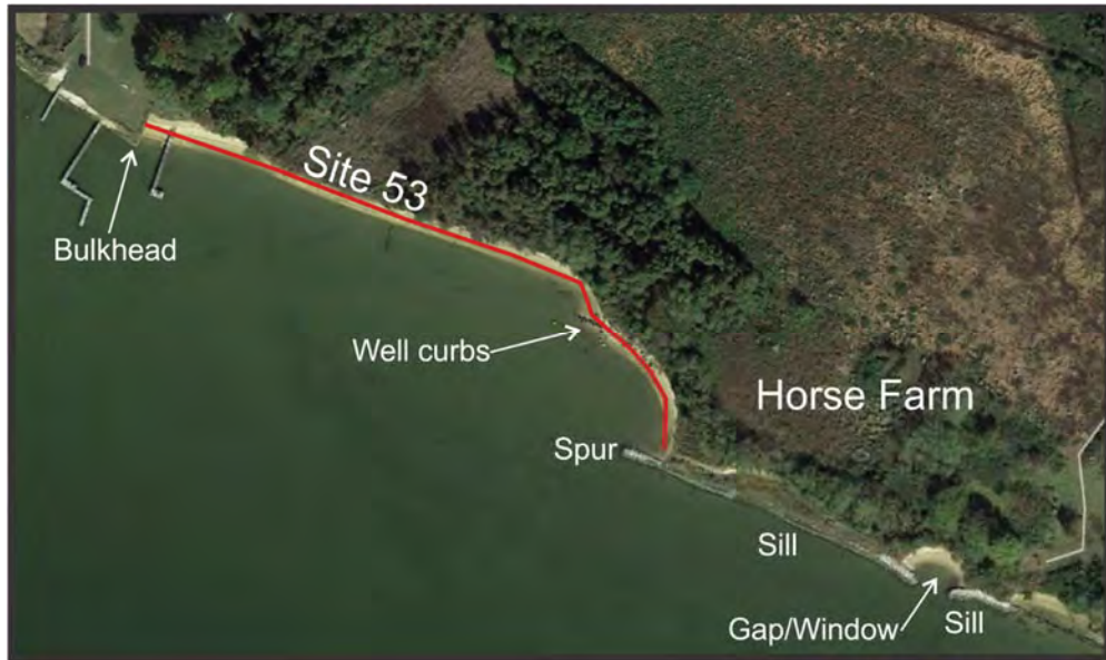
Figure 6-8. Horse Farm shore protection consists of two sills and a spur. The spur and the upriver bulkhead can be considered headlands that define an embayment along the shoreline which will erode to a dynamically stable planform over time.
