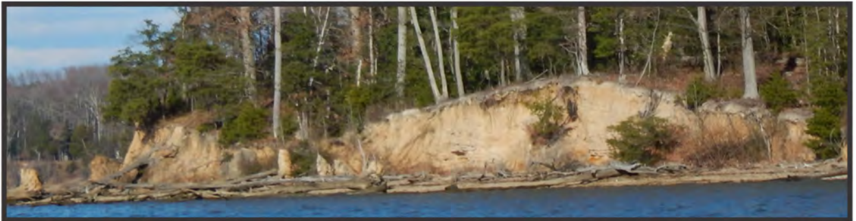
Figure 9-4. Eroding headland at Douglas Point, Site 123, recommend a Type 4 sill.
