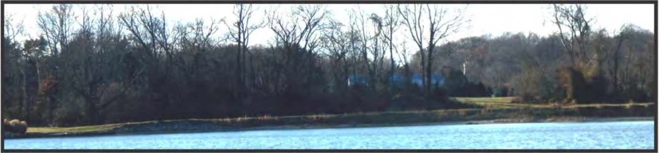
Figure 7-10. West side of Tobacco River with very low eroding agricultural banks, Site 92, recommend Type 3 sill.
