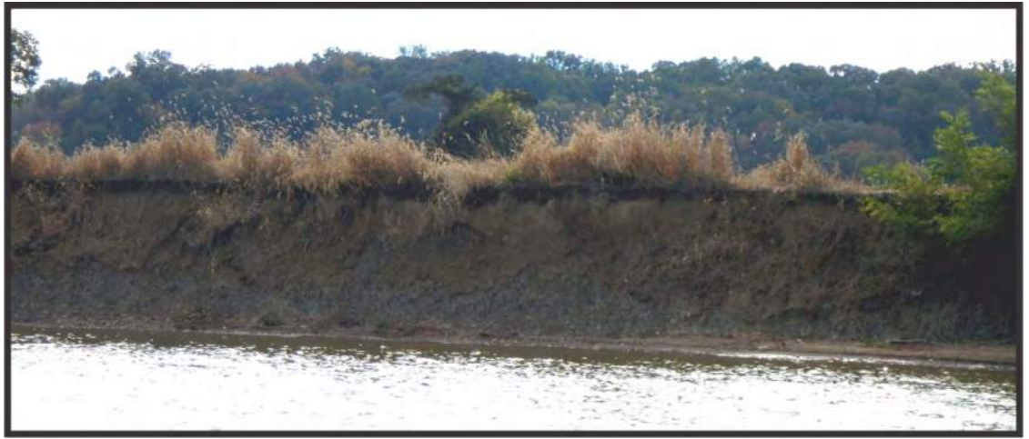
Figure 5-3. Reach 1-A – Eroding agricultural upland bank with no wooded buffer, Site 12, Type 2 sill.
