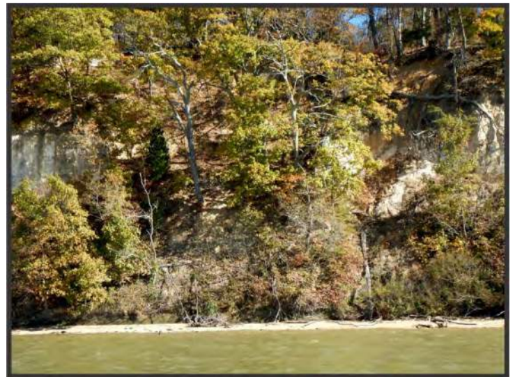
Figure 2-3. Sloughed/slumped material along a high bank. The material protects the base of bank until it erodes.
