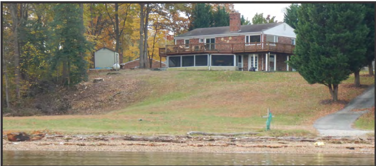
Figure 10-3. Graded banks with a wide backshore can work along some segments of Reach VI-B.
