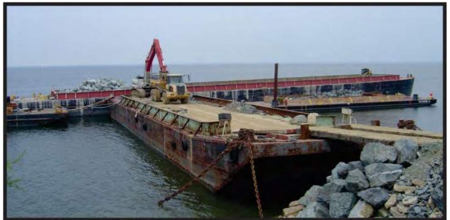
Figure 12-3. Materials being brought to the site by barge.
