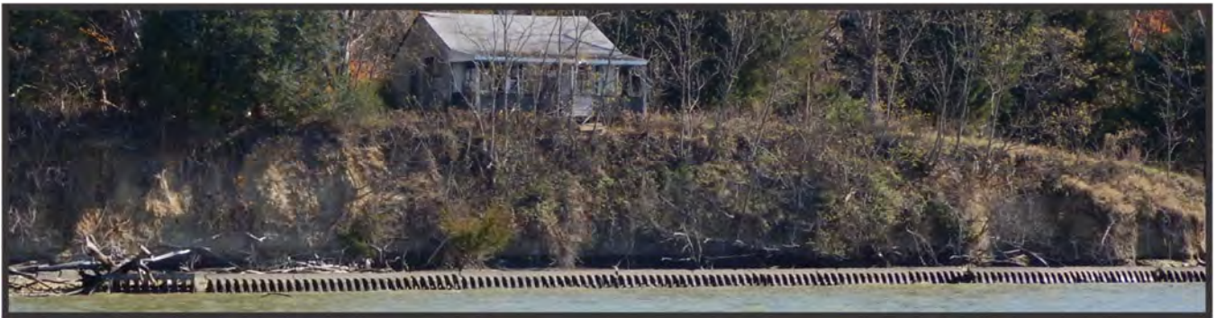
Figure 7-8. Beach prisms along the shoreline are not effective at shore protection.
