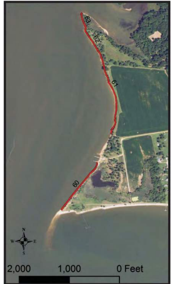
Figure 12-2. Reach II, example of combining Sites 61 and 62 for cost effective design permitting and construction.
