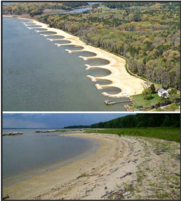
Figure 4-7. Swan Point breakwaters Top: post-construction, pre-planting, 27 March 2012; and Bottom: Four years post-construction, July 12, 2016.
