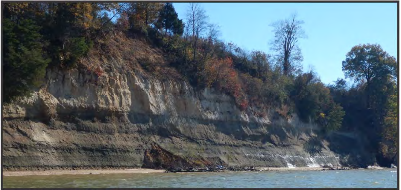
Figure 7-5. High upland bluffs with erosional BOB and bank face with residential land use. Site 76, recommend Type 5 sill.
