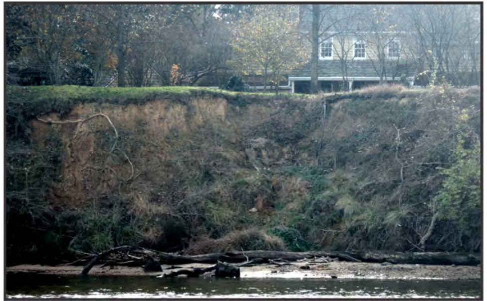
Figure 10-8. Eroding upland near the upriver boundary of Reach VI-C. It is the location of Site 157. Nearshore sill or revetment is recommended due to deep nearshore and historical presence of SAV.
