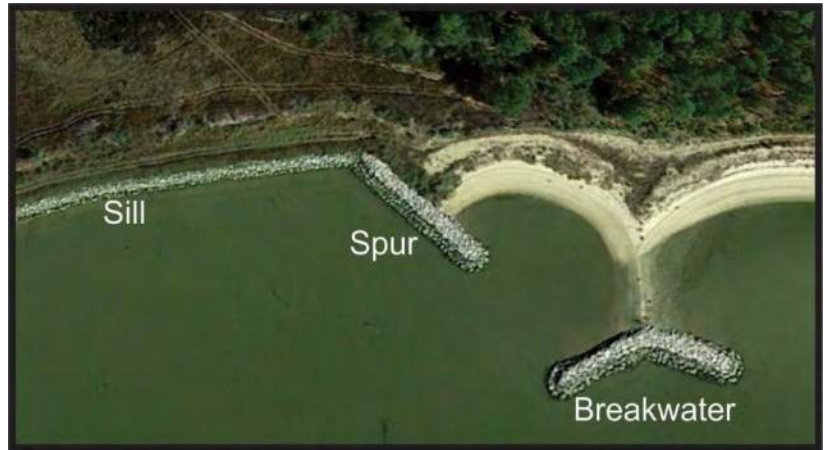
Figure 4-5. Structures at Swan Point include a breakwater, spur, and sill. The spur is attached to the mainland and protrudes at an angle. Google Earth Image.
