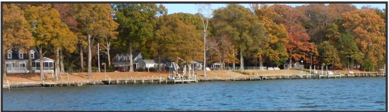
Figure 6-2. Woodland Point residential coast mostly hardened with bulkheads.
