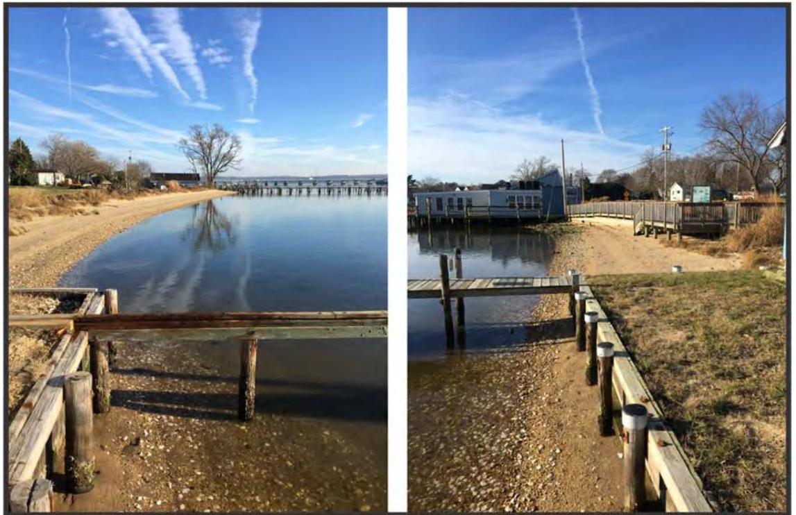
Figure 11-2. Town of Benedict shoreline that is mostly hardened which form some headlands with pocket beaches in between.
